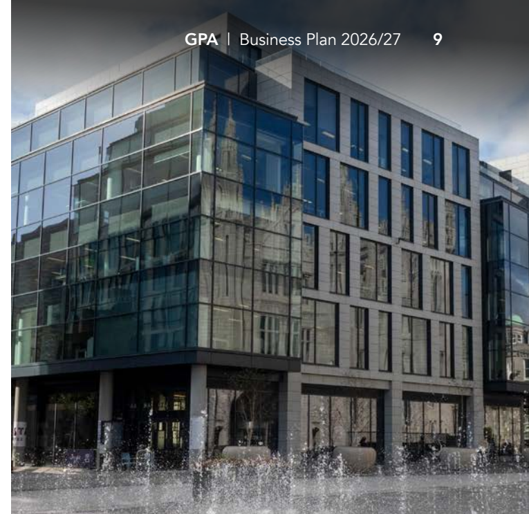
Aberdeen, Marischal Square offices for Great British Energy.
